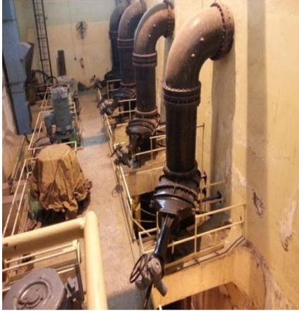
**The Challenge in carrying out the work was that these valves were installed in a vertical Pipe line and the locations of these valves were about four meters above the floor level and the floor level was around 15 Meters below the ground level. The weight of each Plug valve was around 6.5 MT and the crane available inside the pump house was of 5.0 MT lifting Capacity and also the working space available was very restricted.**
