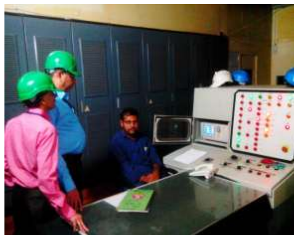
MCGM team witnessing Power readings
